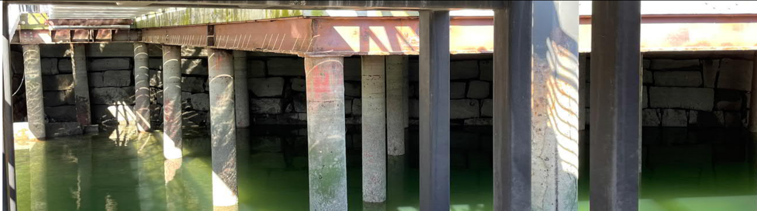
A – View of seawall
