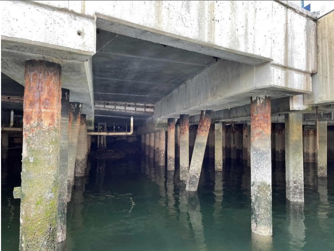
B – View of Pier Structure
