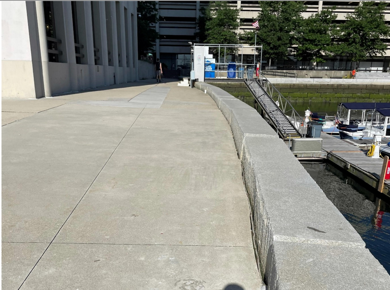
H – View of seawall (North edge)
