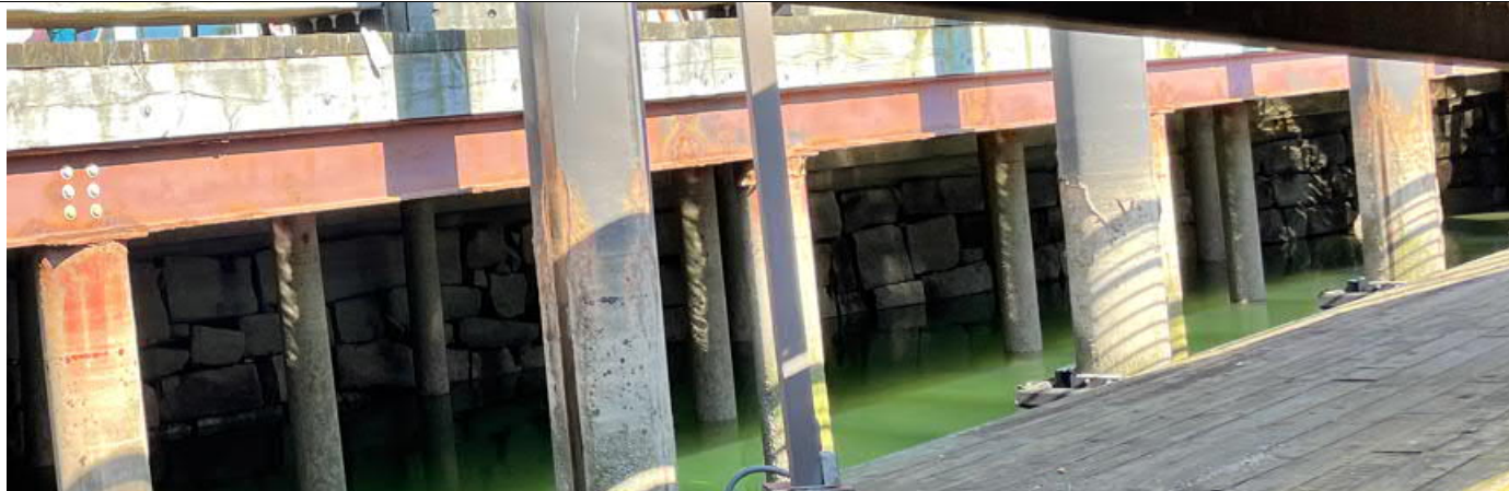
B – View of seawall
