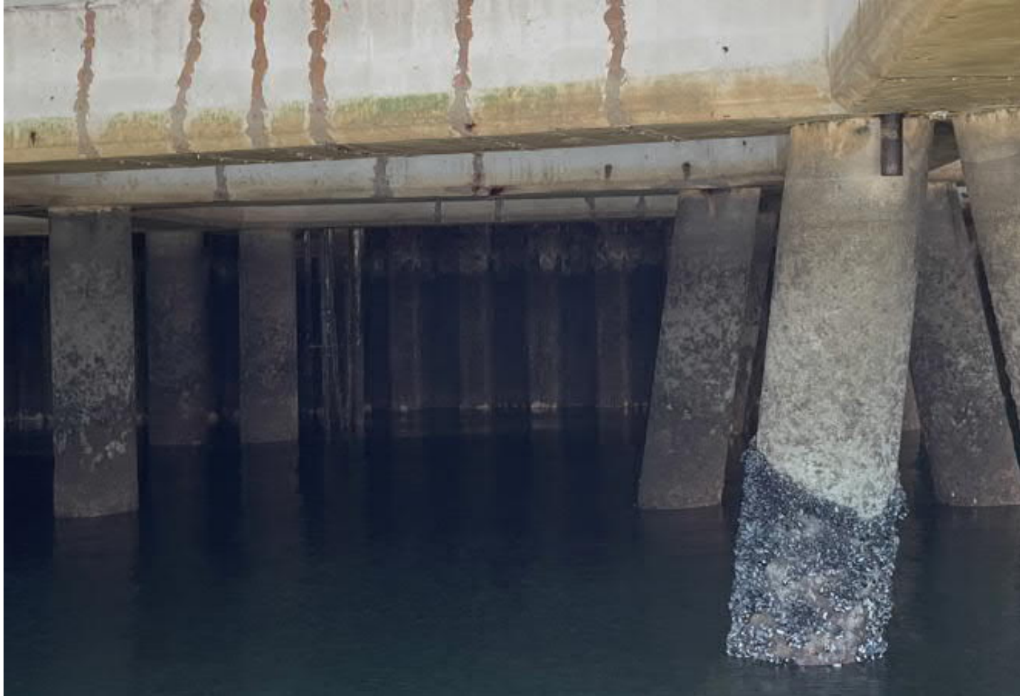
B – View of deck and sheet pile wall
