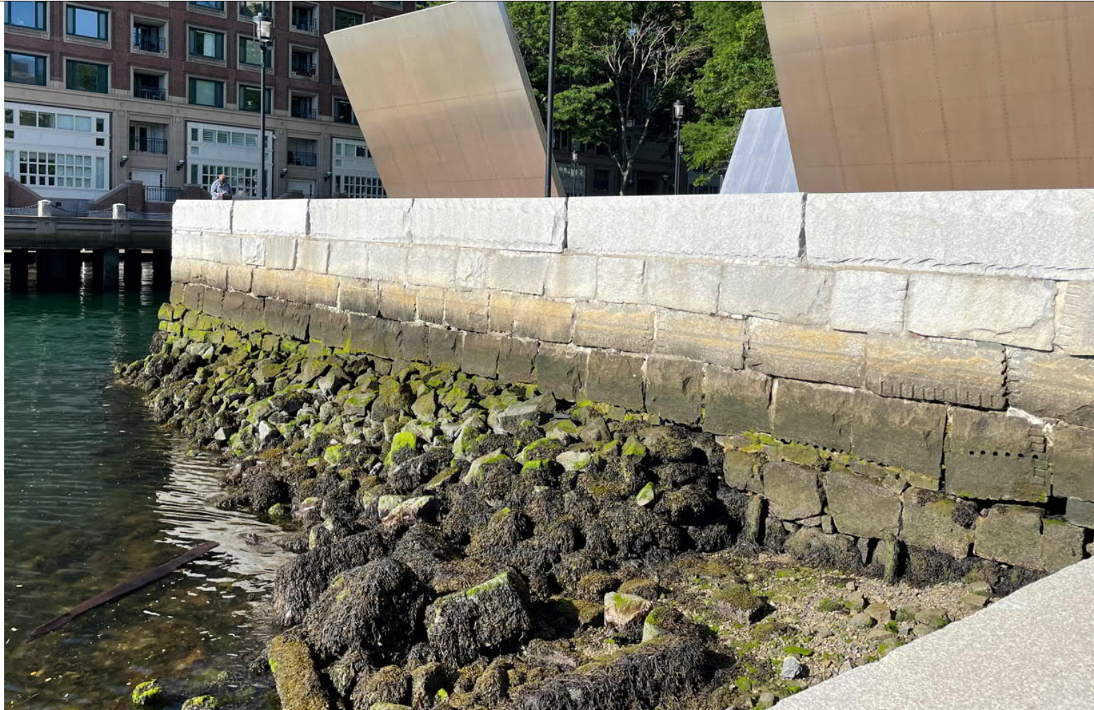
C – View of seawall (location 2)
