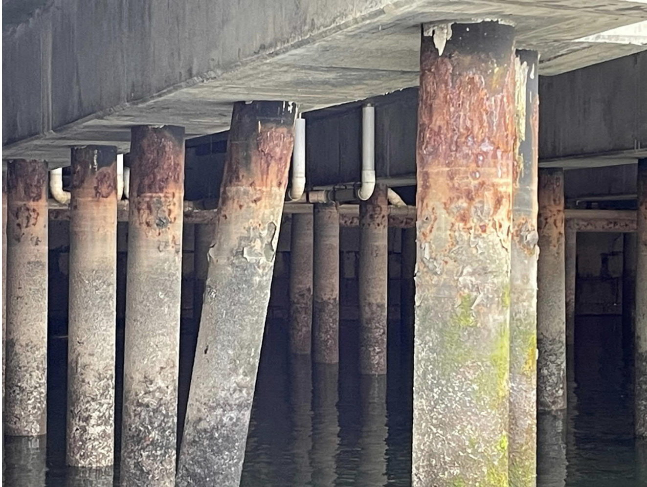
C – Pier support detail view showing condition of piles.
