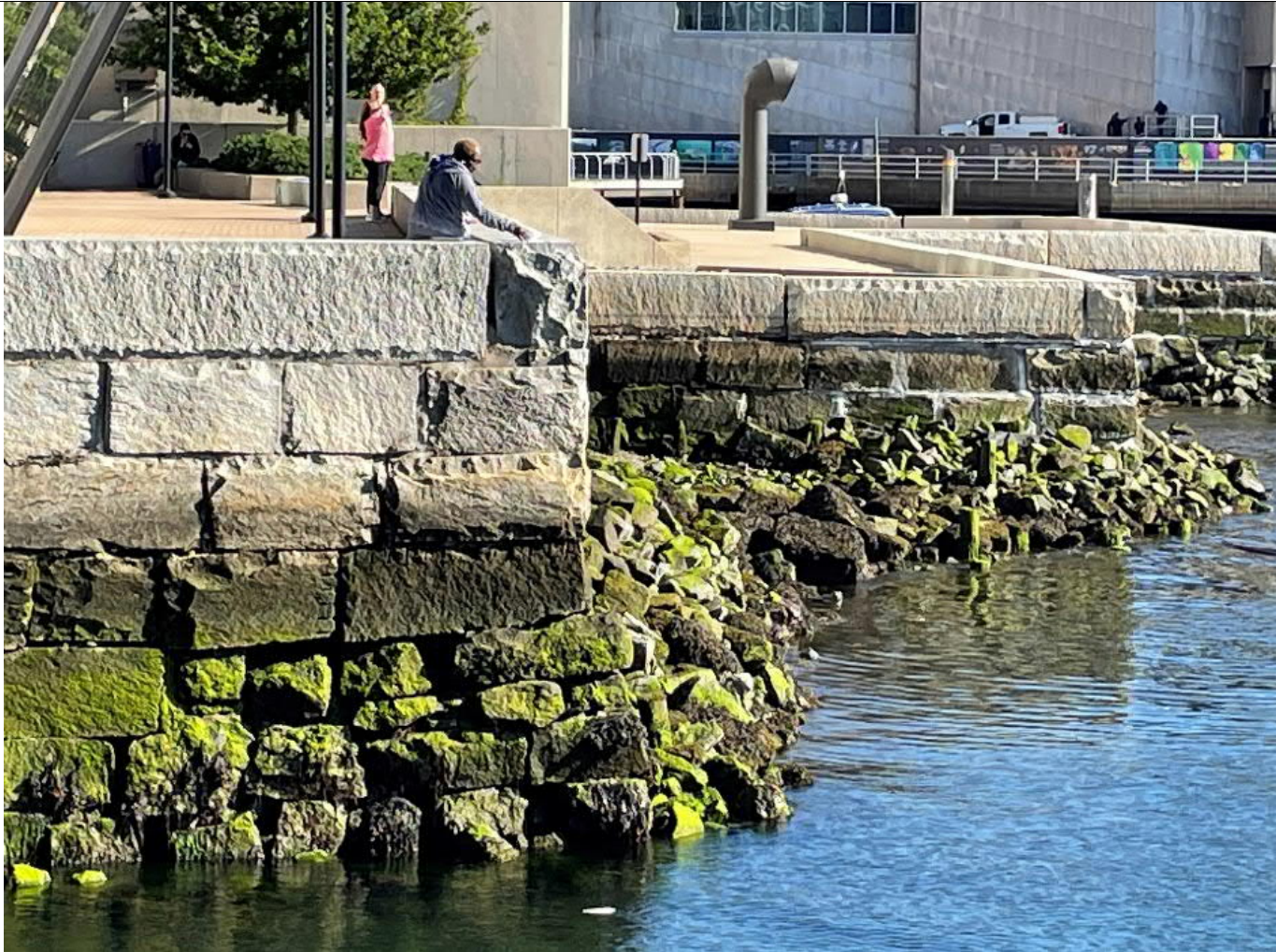
B – View of seawall (location 1)
